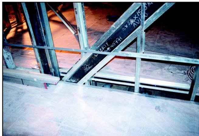
**Figure 2: Gap where a structural wall extends to the slab.**
