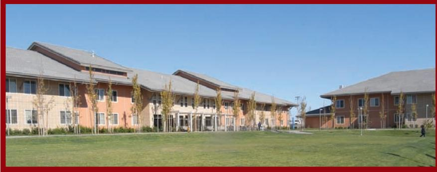
Roof overhangs were optimized for solar shading the fenestration.
