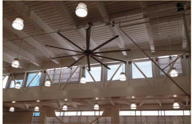
In the great room, louver/dampers provide a relief path for the cool tower, while ceiling fans provide additional cooling.
